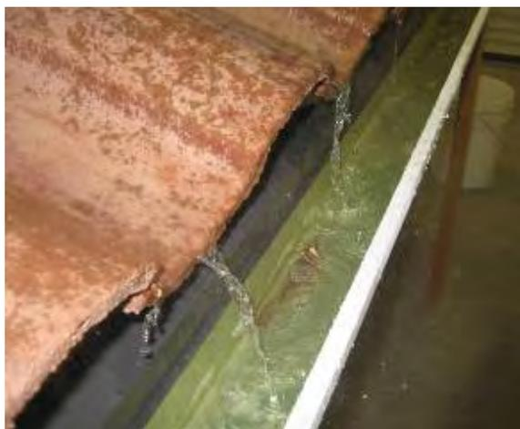
This method works for any tile profile and provides the opportunity to recess the first course of tile up to four inches. This method may also be used in snow areas to prevent the formation of icicles although, in severe winter areas, it may be necessary to further recess the first course and use a wider drip edge.
