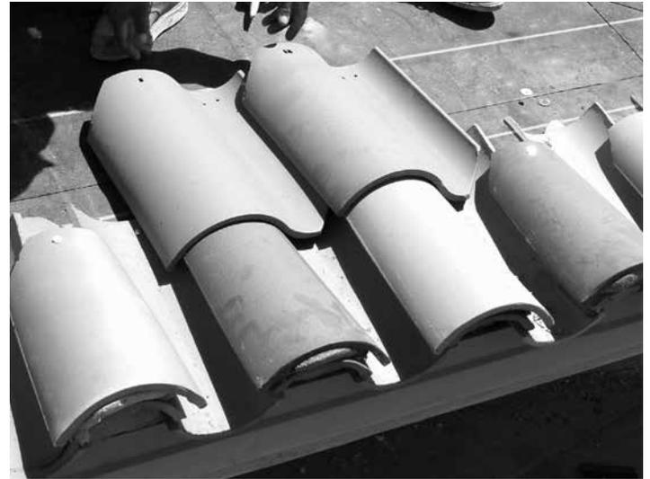
11. Install the 1-Piece "S" Tile or Claylite® tile directly over the top edge of the 2-Piece Mission eave treatment. Ensure that a minimum 3" headlap is maintained.
