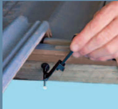
Position clip at 10° angle away from tile edge
