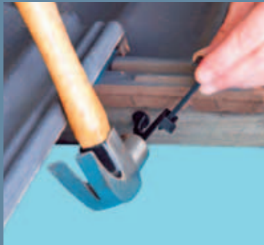
Hammer nail into batten
