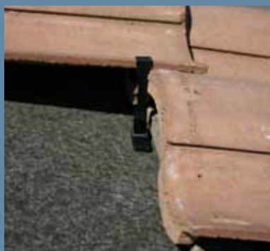
Tall clip on the high profile concrete tile
