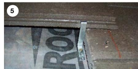
B. Fasten the Wind Clip to the roof deck with a screw or nail through the hole closest to the tile.
